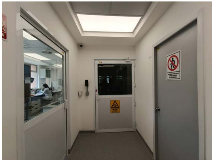
The control room is on the right behind the door marked as "Entry forbidden to unauthorized person".
